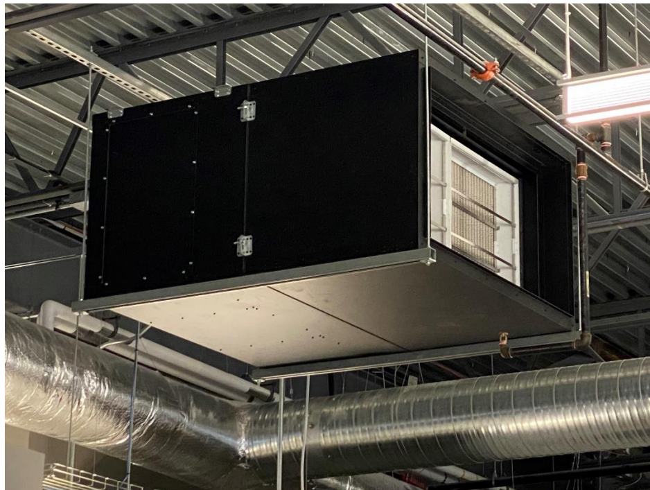
Figure 3: Installed SecureAire Recirculating Fan-powered Unit
